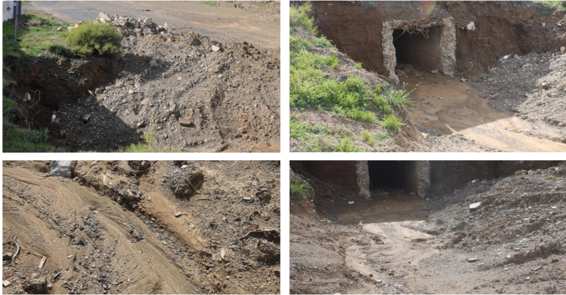
Figure 9-3: Culvert 1 observed onsite with evidence of moisture emanating from the most recent rains. The first culvert is placed on unnamed tributary.
